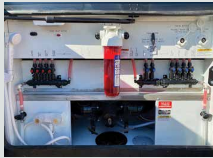
WATER MANIFOLD SYSTEM OFFERING POINT TO POINT CONNECTIONS, EQUALIZED WATER PRESSURE AND TEMPERATURE, AND THE ABILITY TO ISOLATE ANY ISSUE
