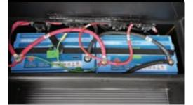
**Dual Low-Temp Lithi**um Auxiliary Batteries (200aH Total)
